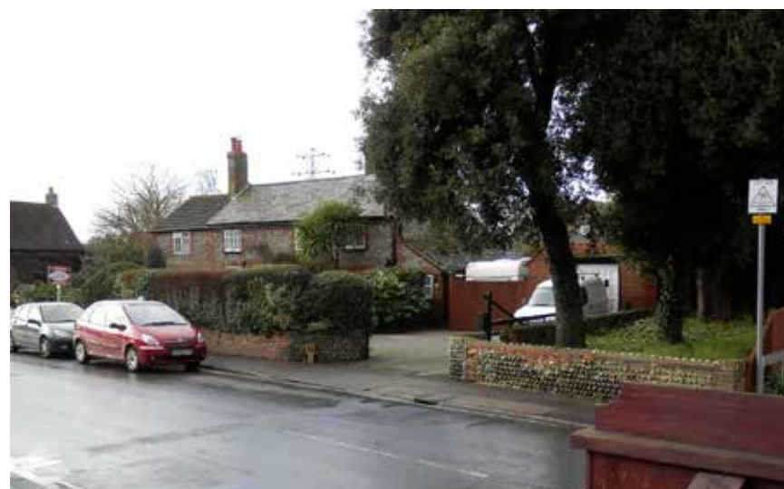
fig. 13: grade II listed properties (west)
